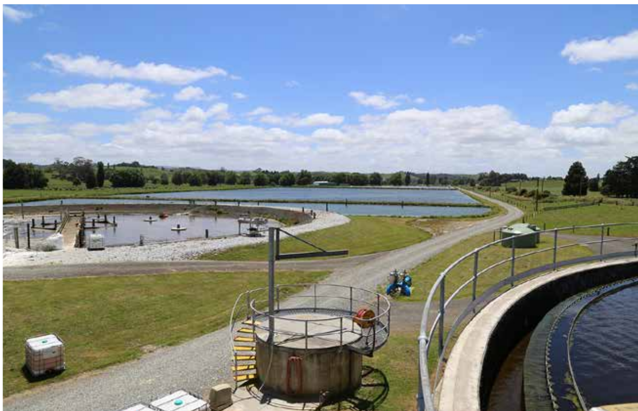
TE KUITI WASTE WATER TREATMENT PLANT
