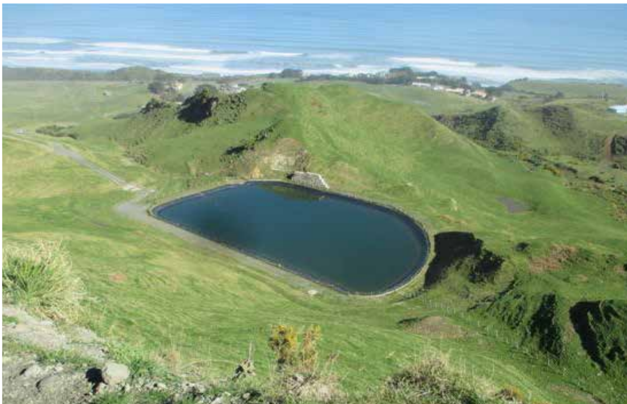
MOKAU WATER STORAGE DAM
